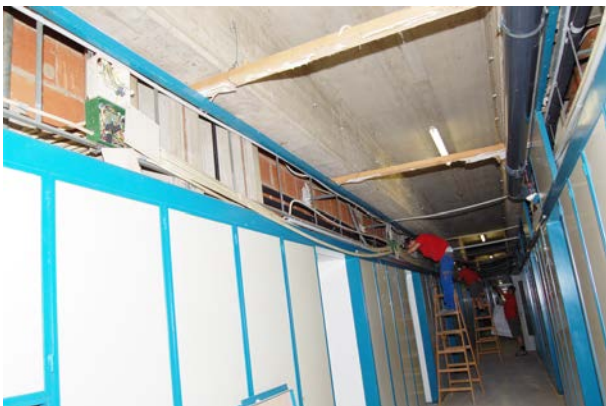
Renovation work on the 2 nd floor.
